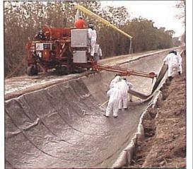
Mobile equipment is used to produce and install the polyurethane fabric lining on site. Installers are trained on the safe handling and use of the material, including what to do in case of a spill.
